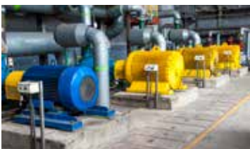
Plant / Equipment Installation
